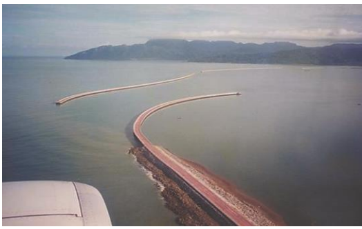
7.0km Offshore Breakwater, Lanagkawi
