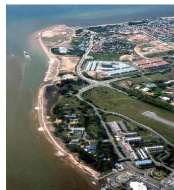
Bintulu Waterfront Protection Works
