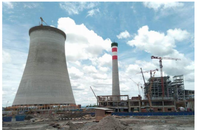
Balingian Coal Fired Power Plant - 2X300 MW
