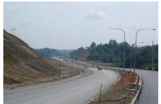
Bintulu Town to Bintulu Airport Dual Carriageway
