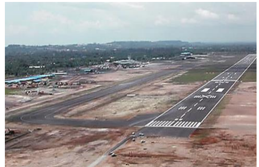
Extension of Miri Airport, Sarawak
