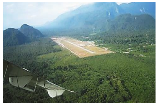
Extension of Mulu Airport, Sarawak
