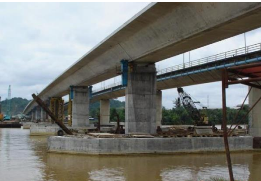
New 2-lane Parallel Btg Kemena Bridge, Bintulu
