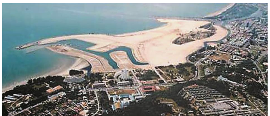
600 Acres of Sea Reclamation for Miri City Extension & Marina Project
