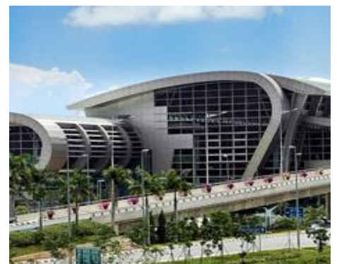
Roof Structure of KKIA Terminal
