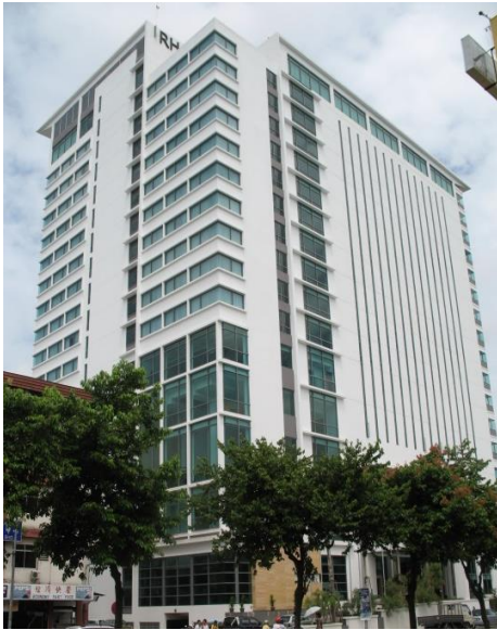
15-Storey RH Hotel Complex, Sibü
