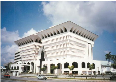
Syariah Court Building Extension. Kuching
