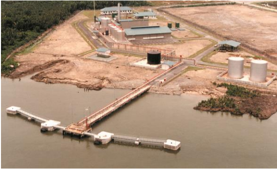
Glue Resin Plant, Kuching
